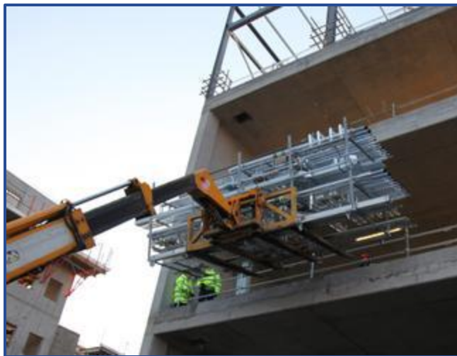
Figure 11: Modular MEP Rack - Courtesy of Google Images
