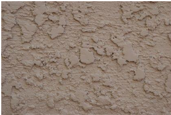
Figure 7: Stucco Exterior - Courtesy of Google Images
